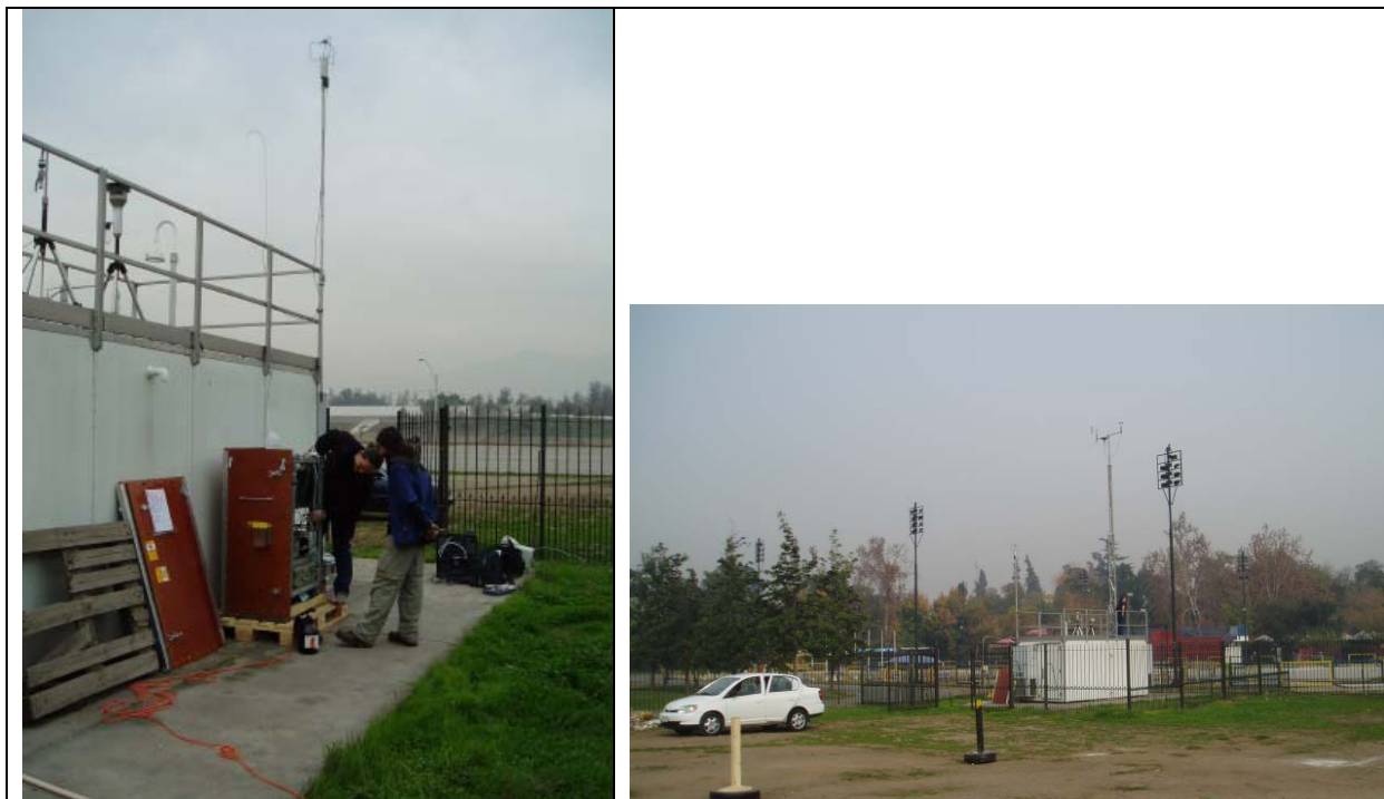
Figure 3. Measurement installations in Parque O'Higgins, Santiago.
